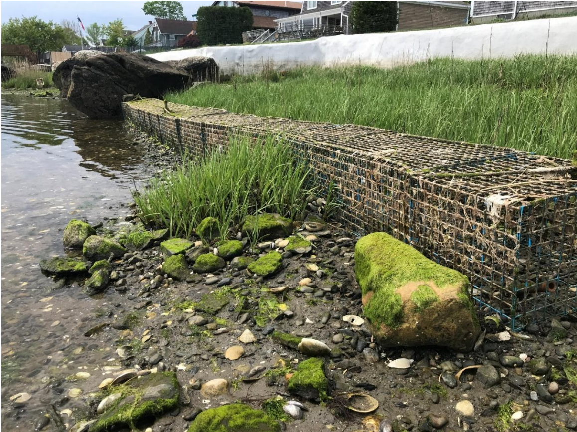
Pilot site in Swansea, MA where 20 structures were placed in front of fringe marsh to reduce incoming wave energy and erosion.
