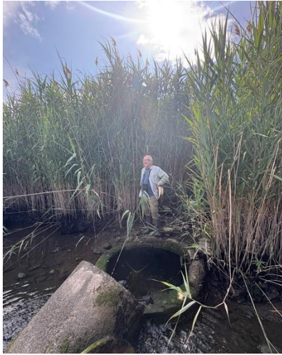
Wastewater outfall surrounded by phragmites at Greenwood
